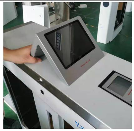
4 Place the turnstile on the position to be installed, press the arrow on the top of the equipment, and place it in the direction of entry and exit. Keep the channel width between 55-58 cm. (Take a tape measure to confirm the width) Keep parallel between the two devices, and reserve power supply And the wire tube or wire groove of the machine wire.
