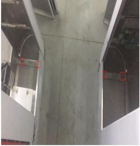
6 Remove the case and punch holes in the marked position with a 12 cm impact drill. (Note: The drill bit must be hit to the end here to prevent the expansion screw from not being able to go down)
