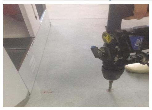
7 After drilling the holes, use a hammer to knock the 10 cm expansion screw into the ground, and then use a 17 wrench to remove the nut, put the case back in place, and lock the nut.
